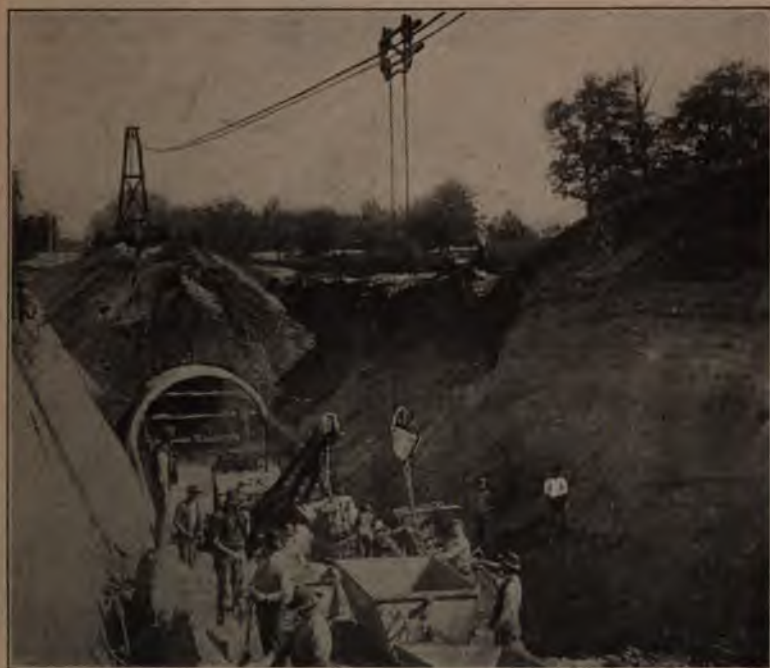
Cableway used on Construction of Large Sewer.
